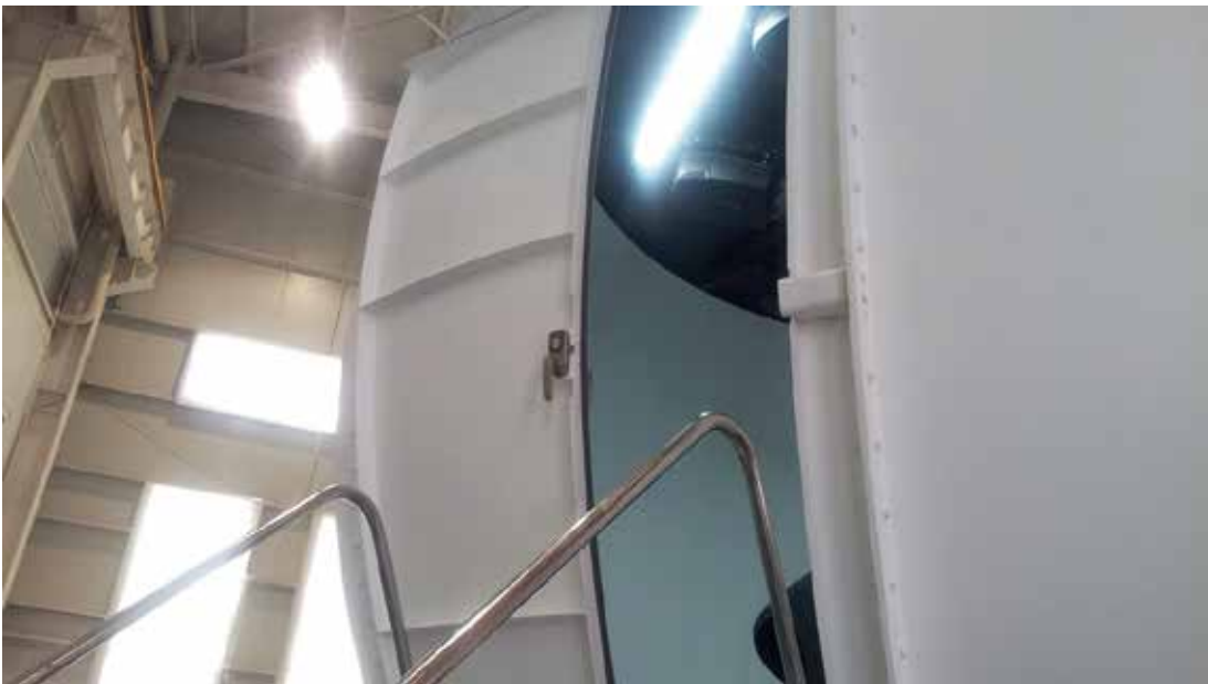
▲Top of the dome (above photo), entrance of the dome (bottom photo)
