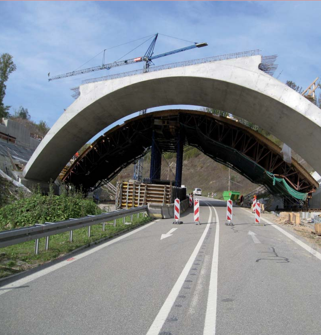
Construction of bridge in Weil am Rhein, Germany
